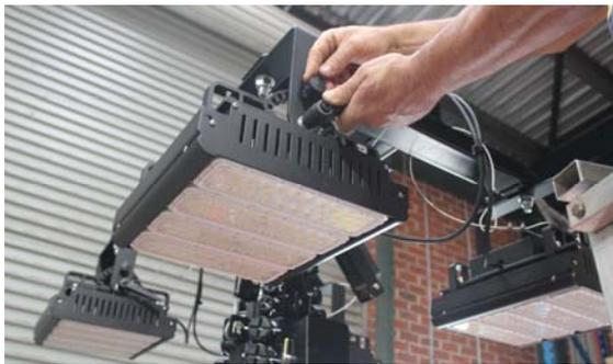
**Fig 1.5.3 LED Light Tilt Adjustment**
